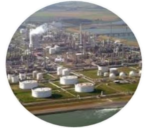
Dow Chemical, Terneuzen
