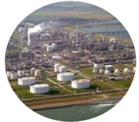
Dow Chemical, Terneuzen
